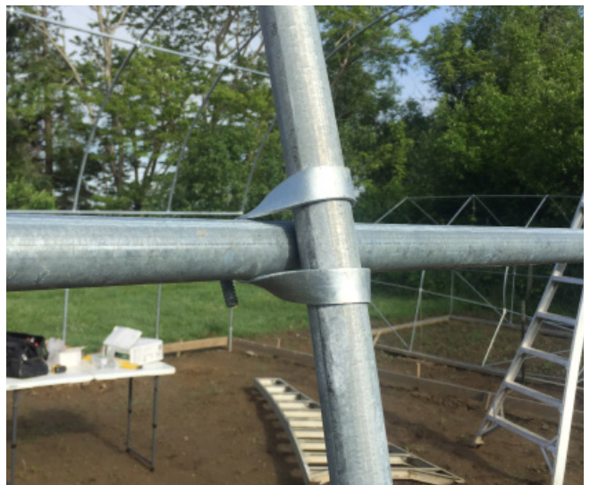
How a purlin clamp connects the hoops to the purlins
