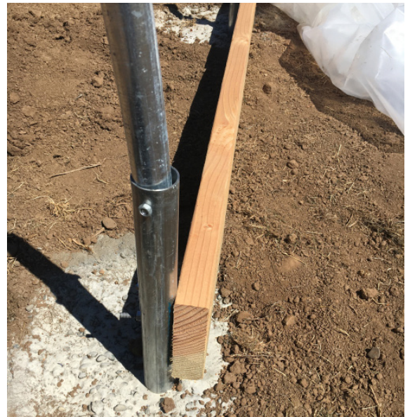
This image shows how a hoop fits into the ground stake. and also previews how the base frame attaches to the ground stake
