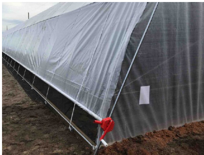
Completed side roll ups. Rolling up nice and straight.
