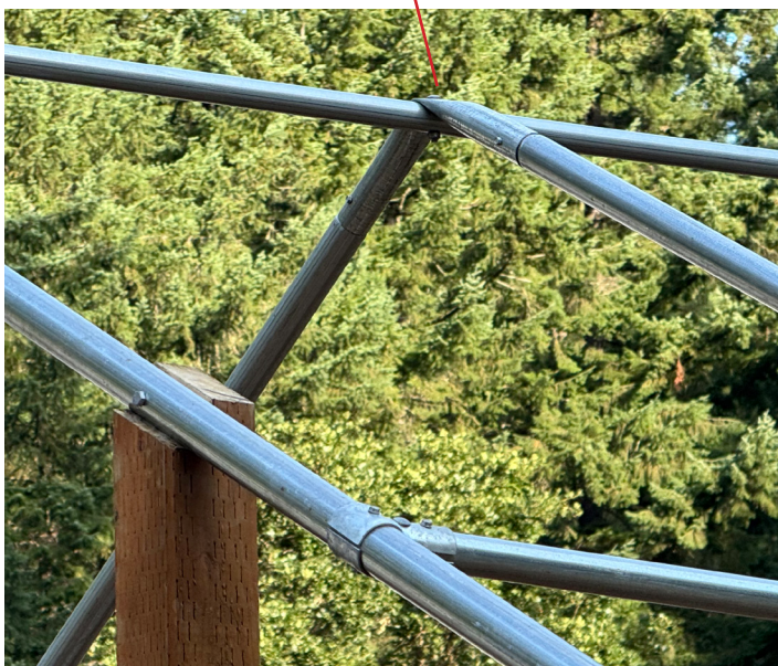
Center purlin attached to the peak connector
